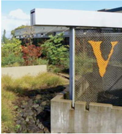
The bioswale at Henry V keeps rainwater from turning into urban runoff.
